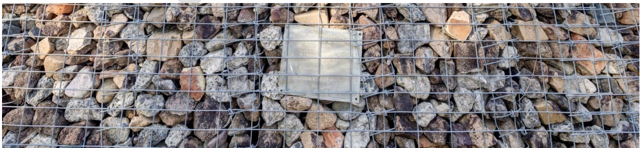
Figure 24: Promoting sustainability by using recycled materials in the Park's gabion walls.
