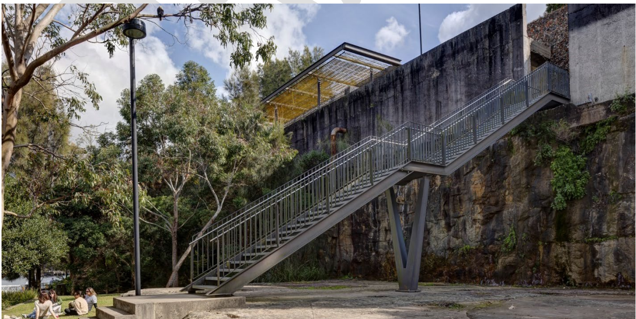
Figure 29: The significant topography of the site makes access challenging in some areas.
