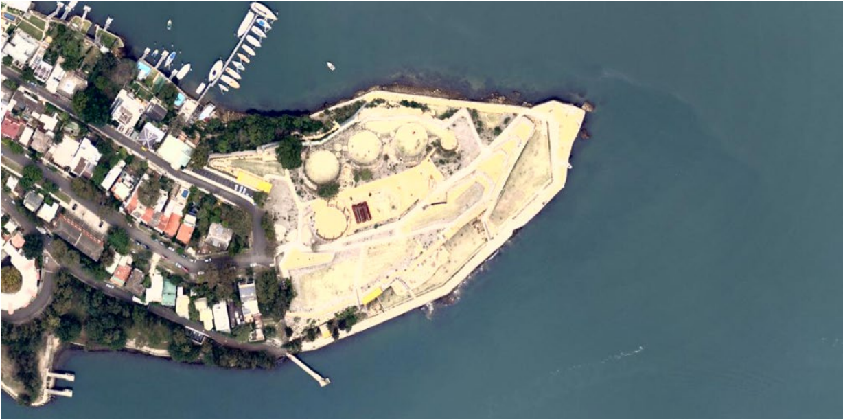
Figure 18: Ballast Point Park 2009. (Source: Nearmap)
