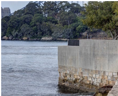
7 Caltex Pilot Jetty remains
