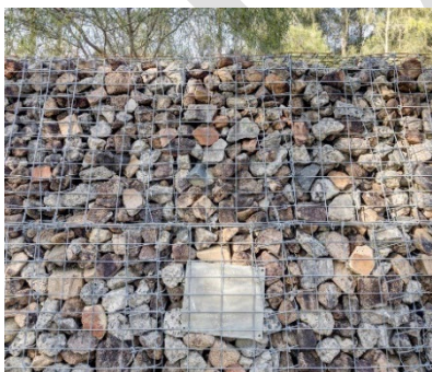
10 Artefacts within gabion walls
