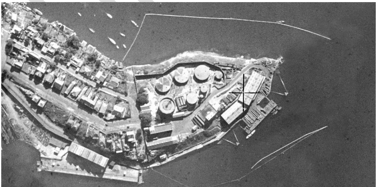
Figure 16: Ballast Point Park 1943. (Source: SIX Maps)
