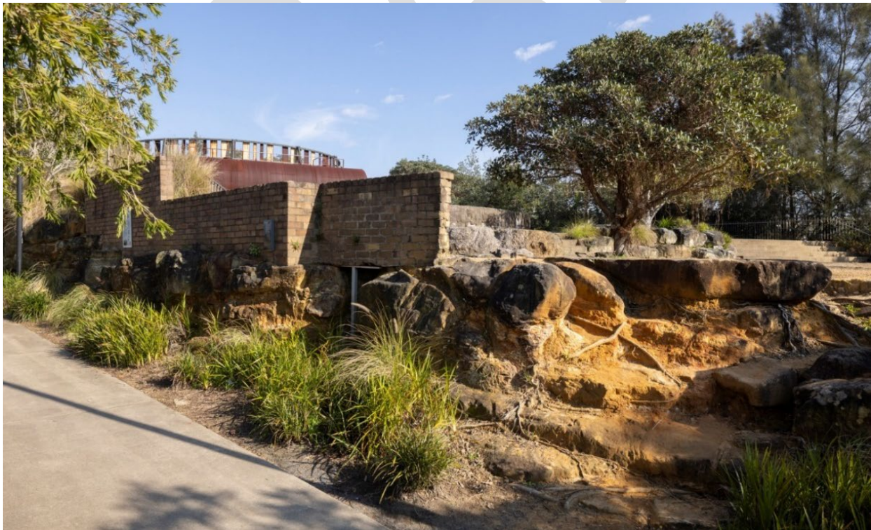
Figure 24: Erosion and run-off affected ridge-top.
