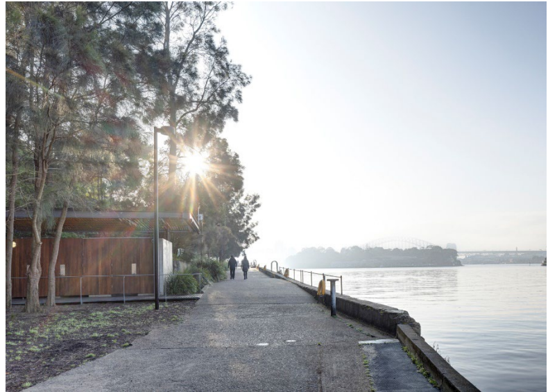
Figure 29: Toilets at the lower park entry.
