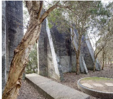
5 Bund Wall (retained portion)
