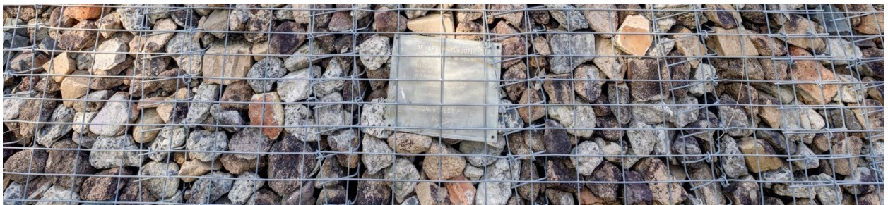
Figure 23: Promoting sustainability by using recycled materials in the Park's gabion walls.
